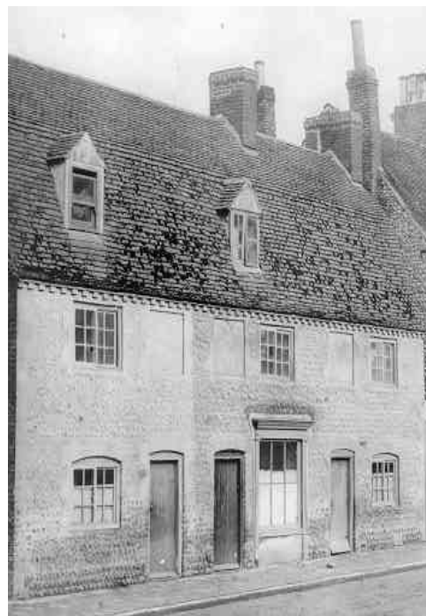
A gambrelled roof with gabled dormers
