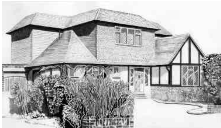
An unacceptable bulky dormer
