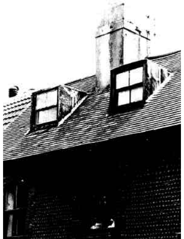
Traditional flat topped lead clad dormer
