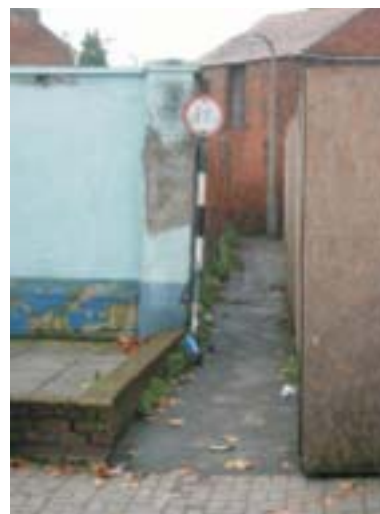
This unattractive footpath link has limited opportunities for natural surveillance, is too narrow, and ends with an awkward turn at the top. As such it has no sense of ownership and provides opportunities for crime and anti social behaviour.
