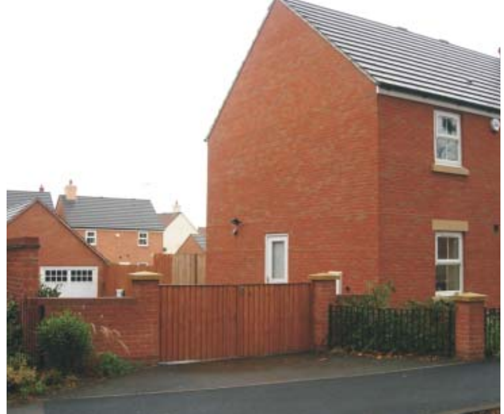
In this development boundary walls at the side of properties, which do not interfere with the potential for maximising natural surveillance, have been constructed to a height which screens the wheelie bin. The addition of lockable gates also provides extra security.
