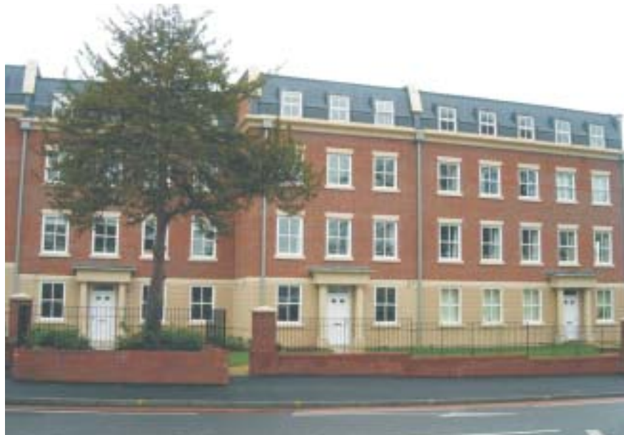
In this recent development the ground floor apartments have all been provided with their own entrances, protected by an area of defensible space. This has helped to promote activity on this front elevation.
