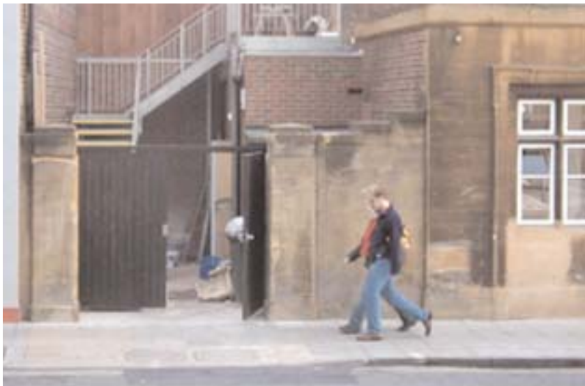
These gates have been used to conceal a bin storage area and provide security to an external staircase however they have not been properly maintained and there is no sense of ownership so they are left open creating an unattractive streetscape.
